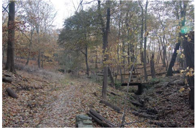
Photo 31. Footbridge over stream near Watson's Trail
