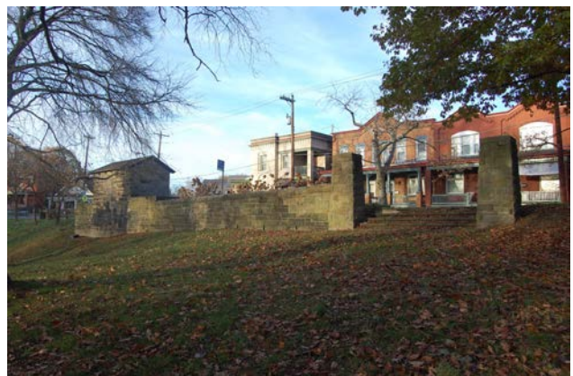
Photo 25. Bus (trolley) shelter ensemble and Leaning Ash trailhead at Perrysville Avenue and Chemung Street, view from park
