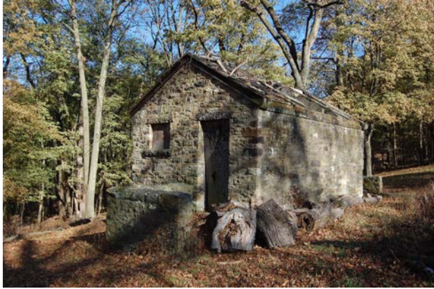
Photo 39. Rest room building at Watson's Cabin camp site
