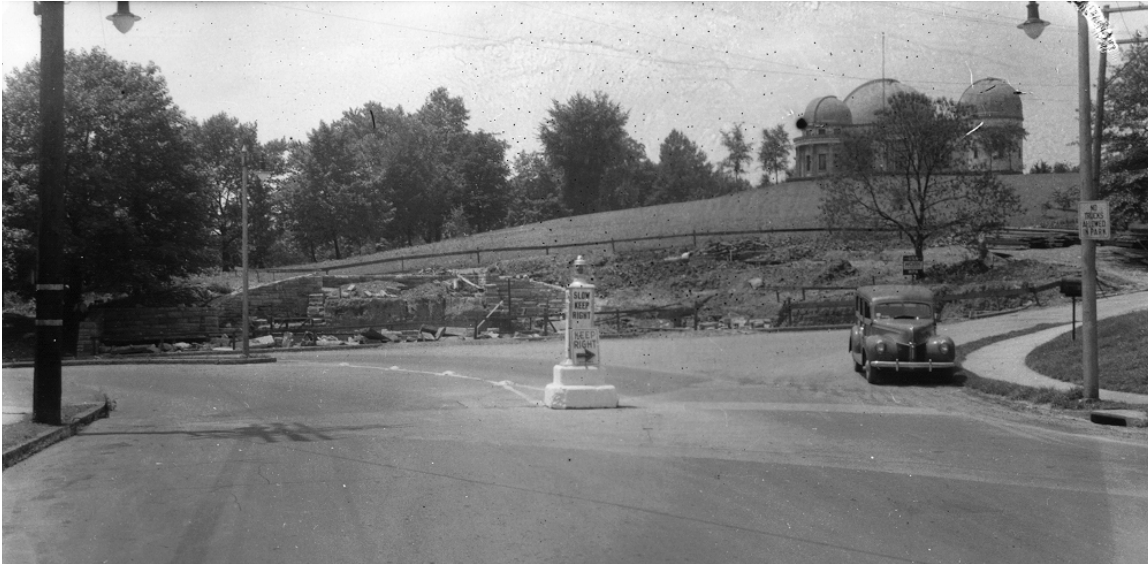
Figure 12. Riverview Avenue entrance under construction, 1940 (Pittsburgh City Photographer Collection)
