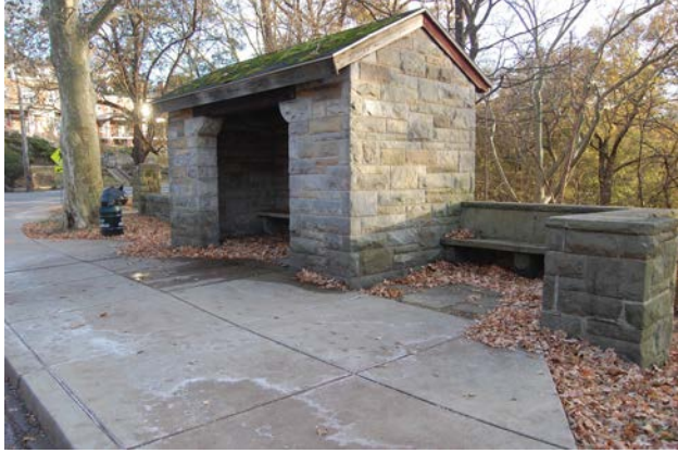
Photo 26. Bus (trolley) shelter ensemble at Perrysville Avenue and Delaware Street
