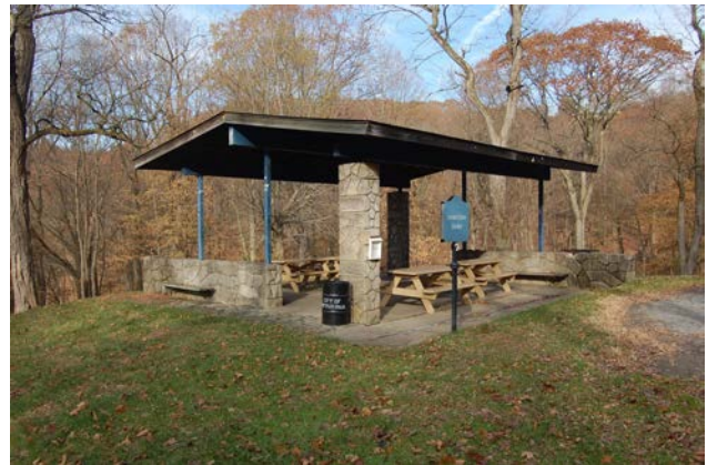
Photo 33. Locust Grove Shelter
