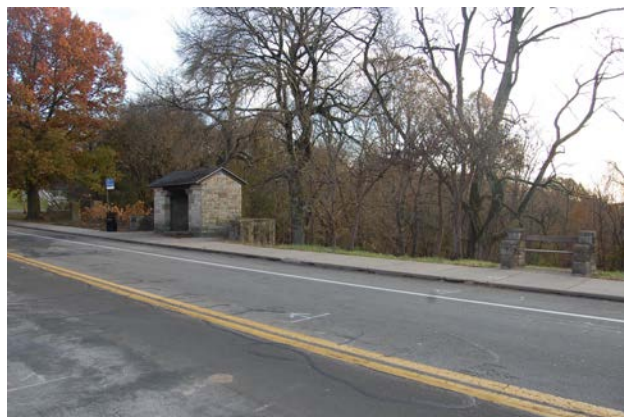
Photo 24. Bus (trolley) shelter ensemble at Perrysville Avenue and Chemung Street
