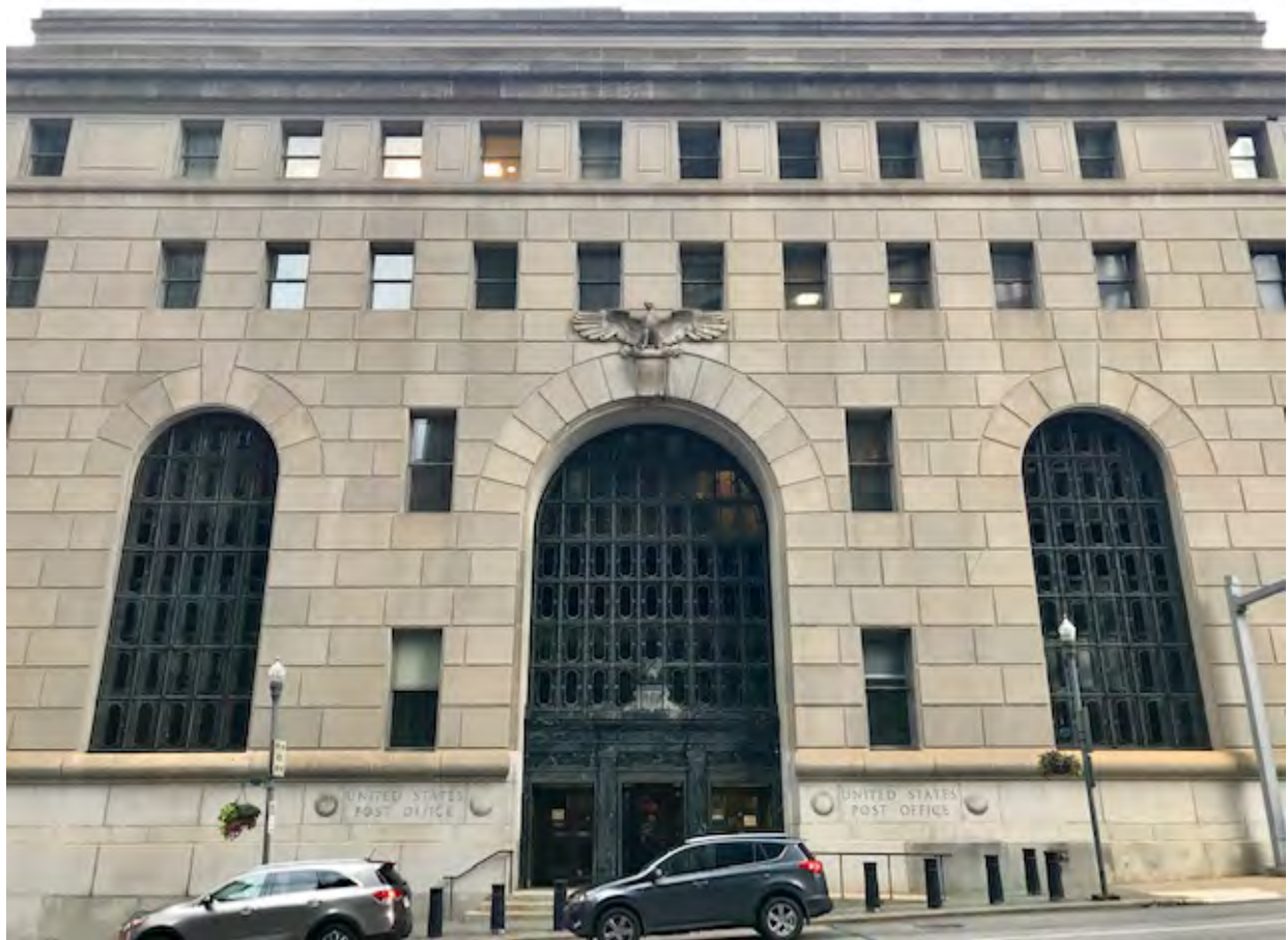
Photo. 4. Weis Courthouse, Seventh Ave. Façade , July 2019. Source: Matthew W.C. Falcone.
