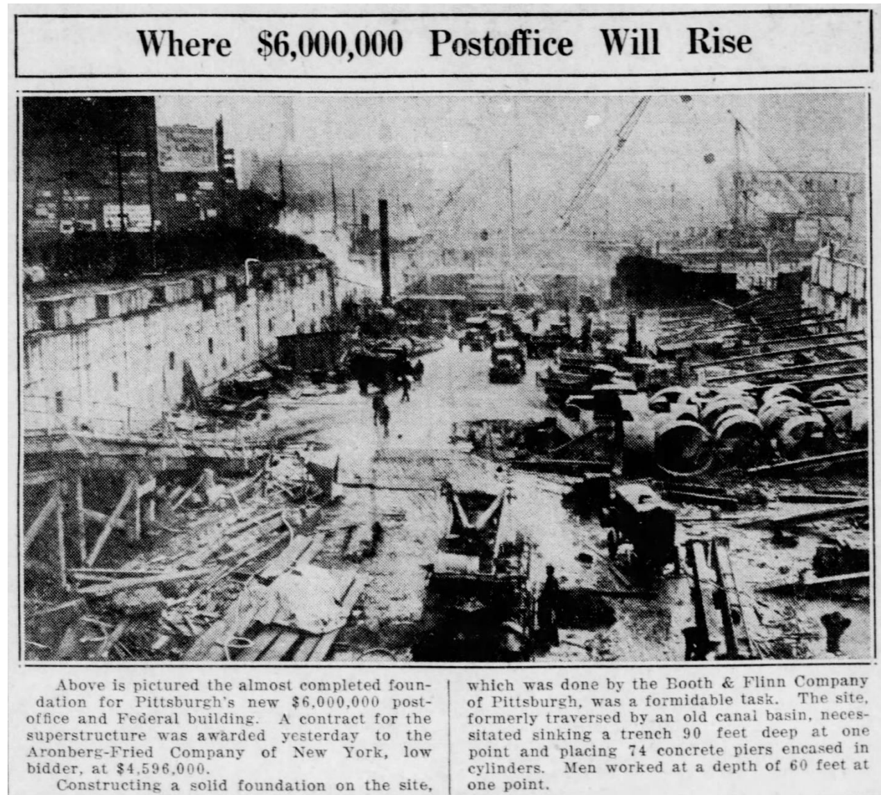
Figure 9. Foundation under construction. Pittsburgh Post-Gazette , December 23, 1931, p. 13.
