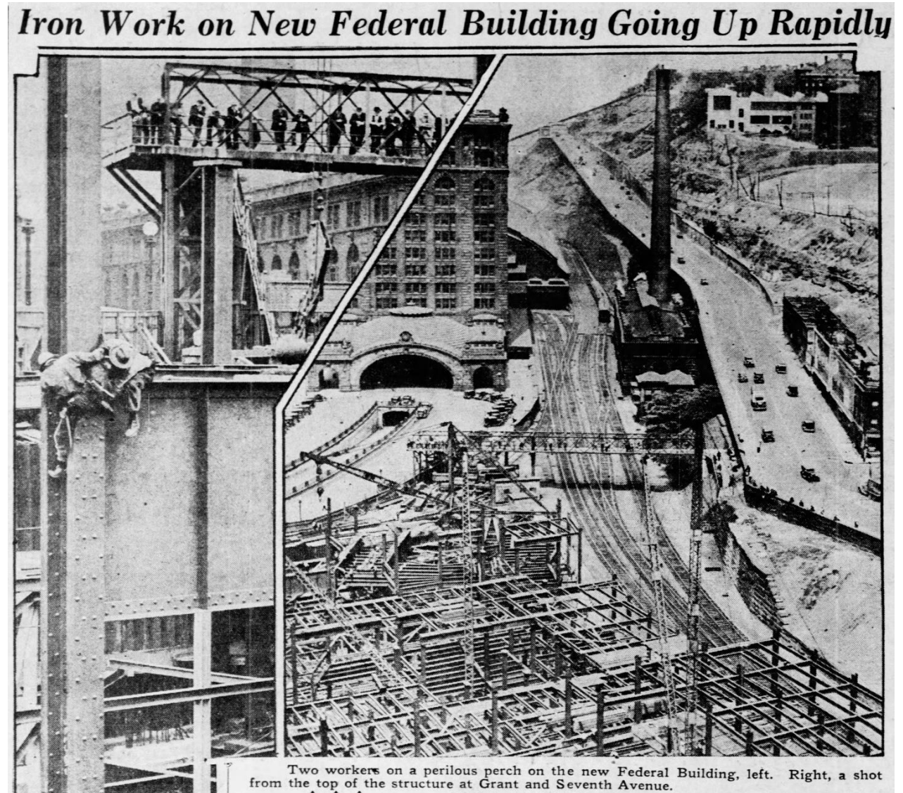
Figure 10. Work progressing on the steel frame. Pittsburgh Press , June 13, 1932, p. 12.
