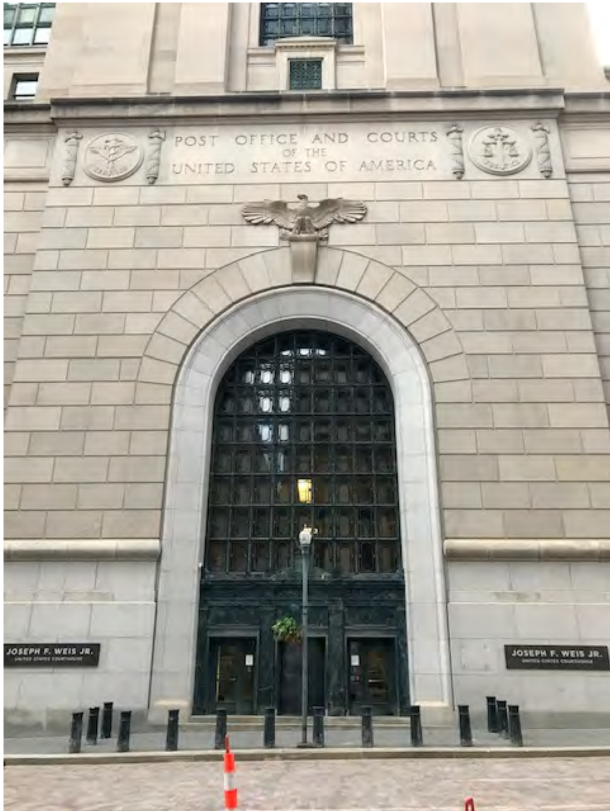
Photo. 2. Weis Courthouse, Grant St. Façade, Main Entrance Detail , July 2019. Source: Matthew W.C. Falcone.
