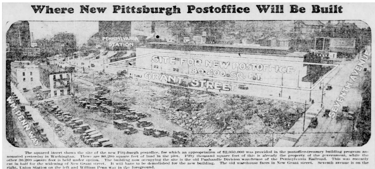
Figure 5. The proposed site after the Grant Street realignment, 1926. Pittsburgh Gazette Times , June 6, 1926, sec. 3, p. 12.
