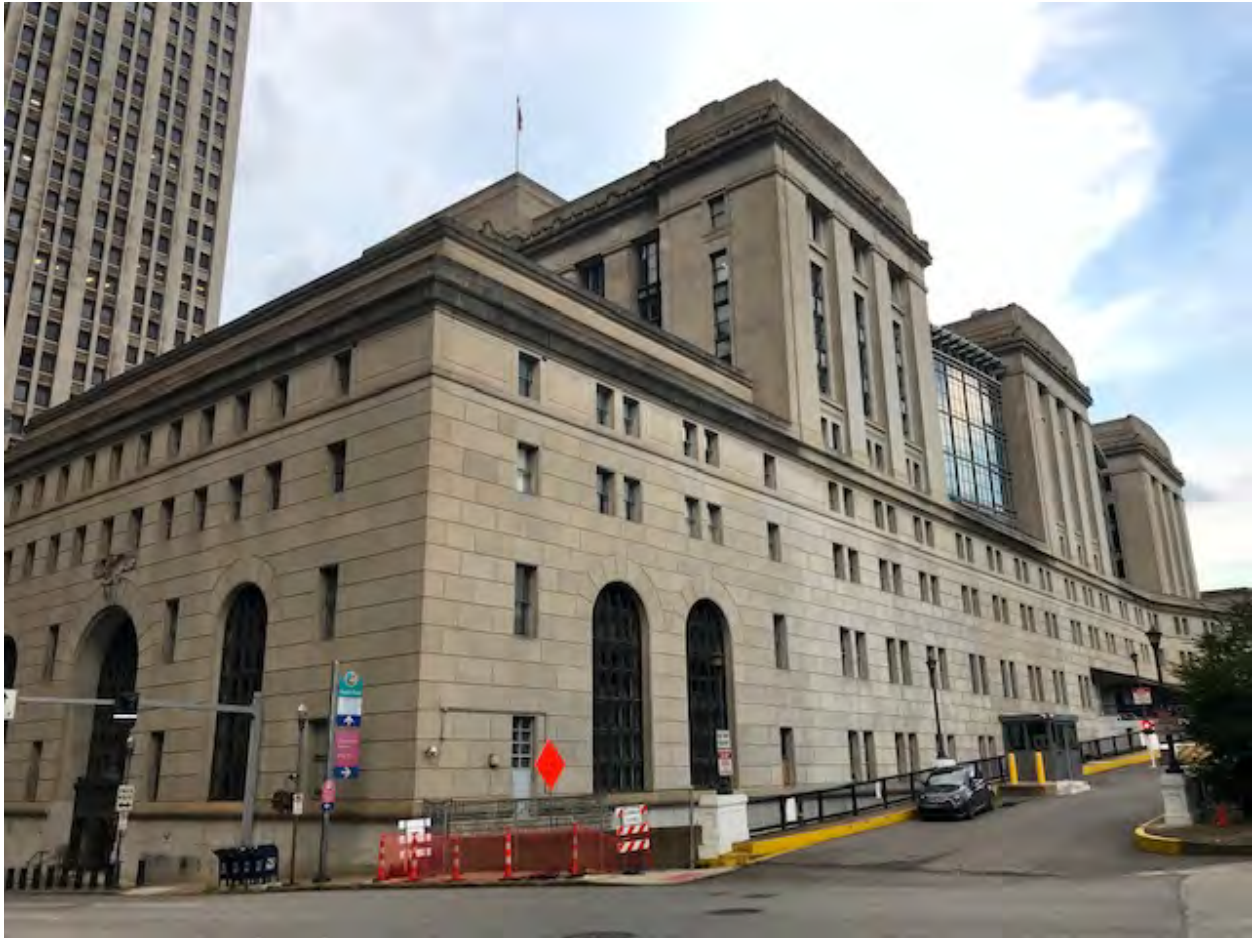
Photo. 6. Weis Courthouse, Seventh Ave. & Bigelow Blvd. Facades , July 2019. Source: Matthew W.C. Falcone.
