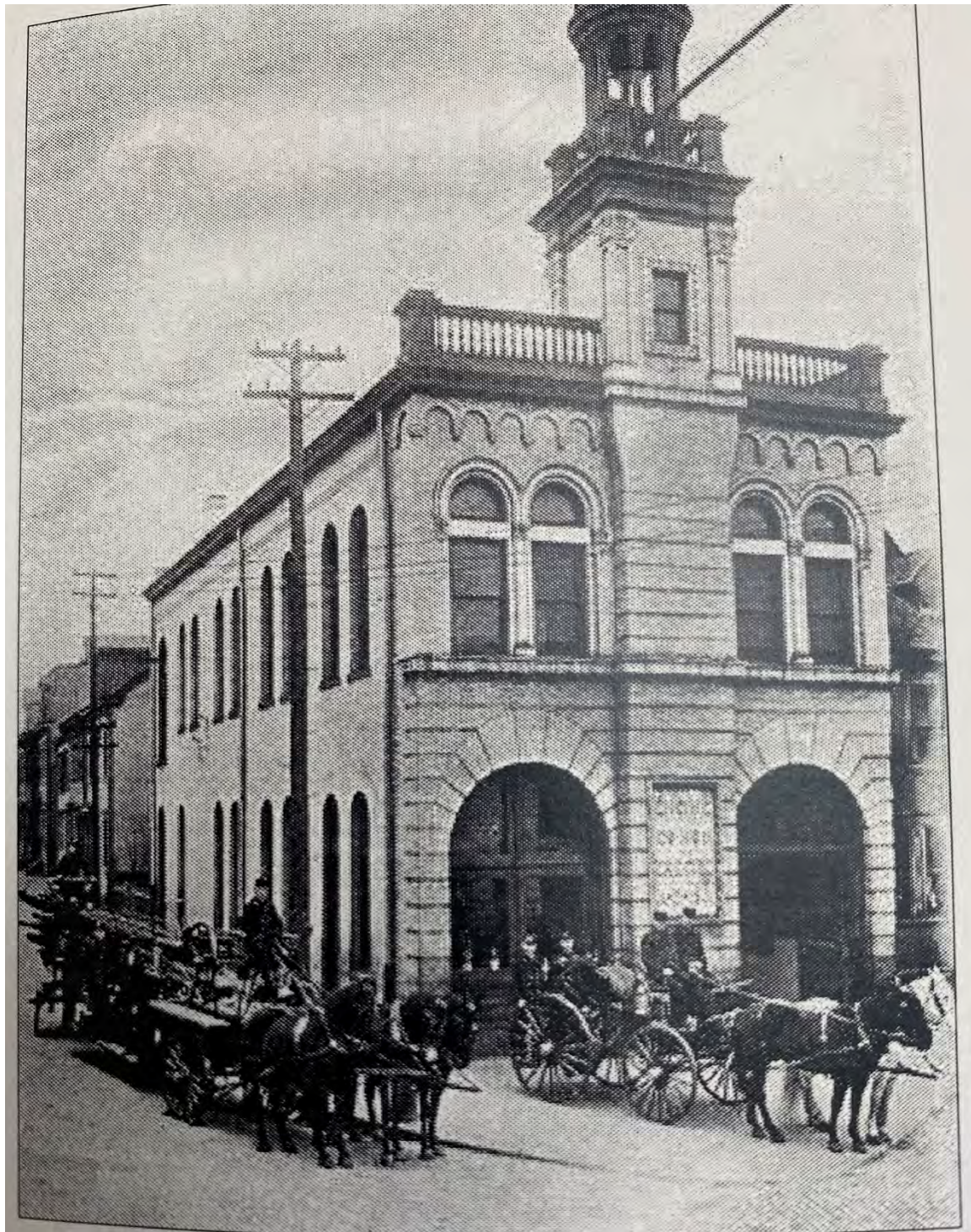
Figure 8: The only known photo of the fire house as it was originally constructed, c. 1901. Note the balustrade at parapet and the cupola on top of the square Italianate tower. Photo courtesy of Footprints of Troy Hill.
