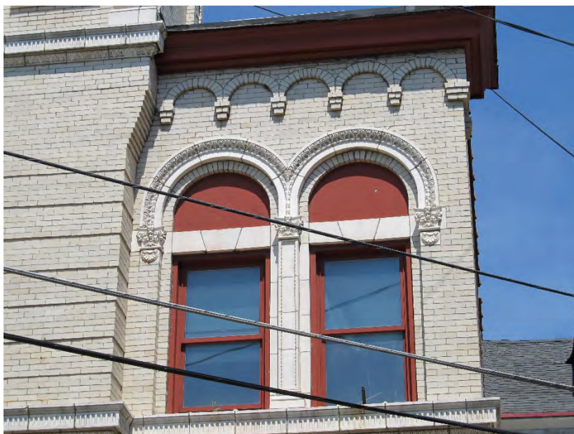
Photo 4: Fenestration detail, southeast (facade) elevation. Amanda Stander, 2020.
