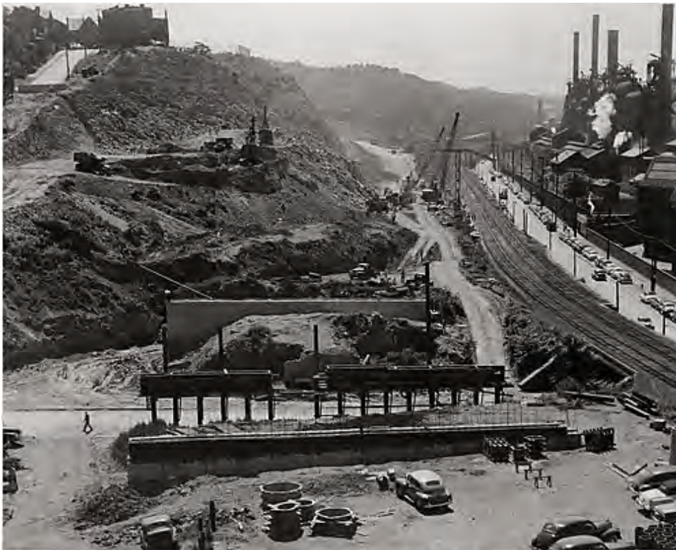
Fig. 4. Nestler, Fran. Construction of the Penn-Lincoln Parkway at Bates Street . 1950. Carnegie Museum of Art Collection of Photographs. Accessed: https://historicpittsburgh.org/islandora/object/pitt%3A85.4.96
