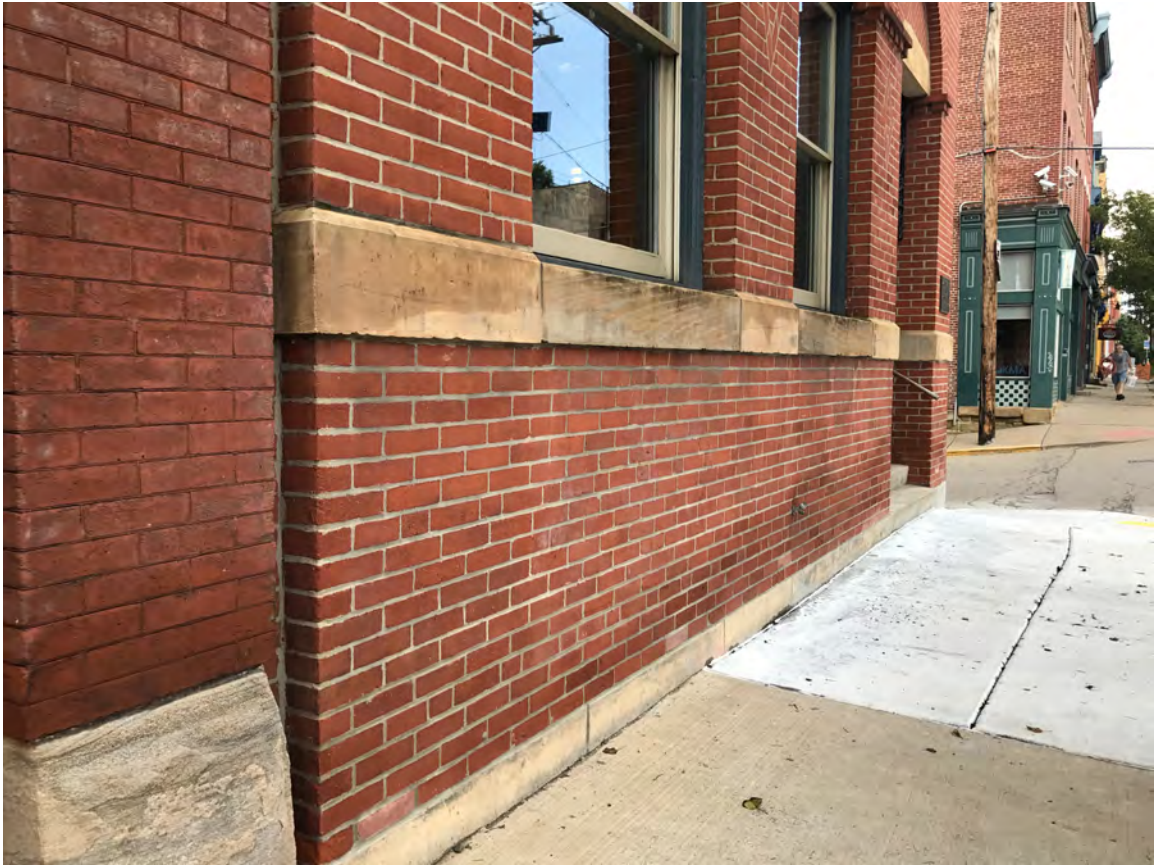
Photograph 8. Brick Work with Stone Trimmings.
