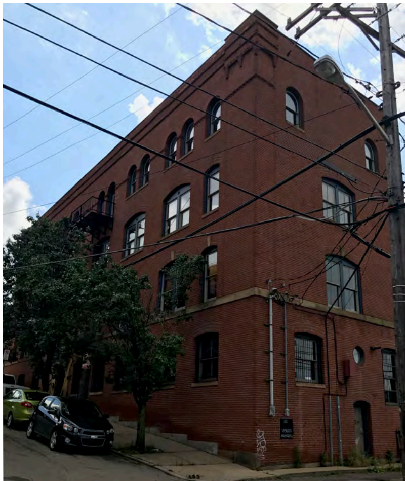
Photograph 4. Side and Rear Elevations. (From Mulberry Way).
