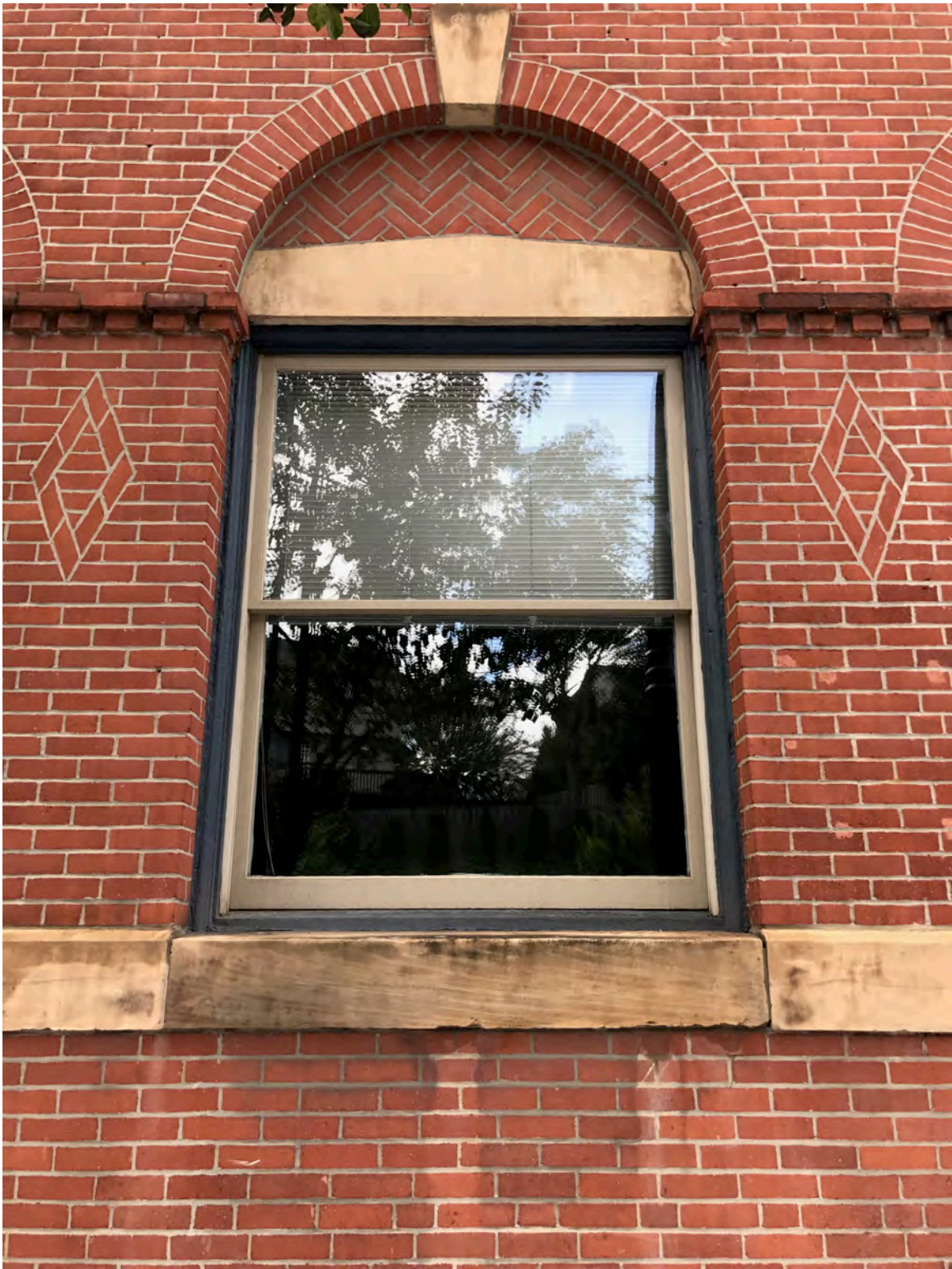
Photograph 9. Ground Floor Window.
