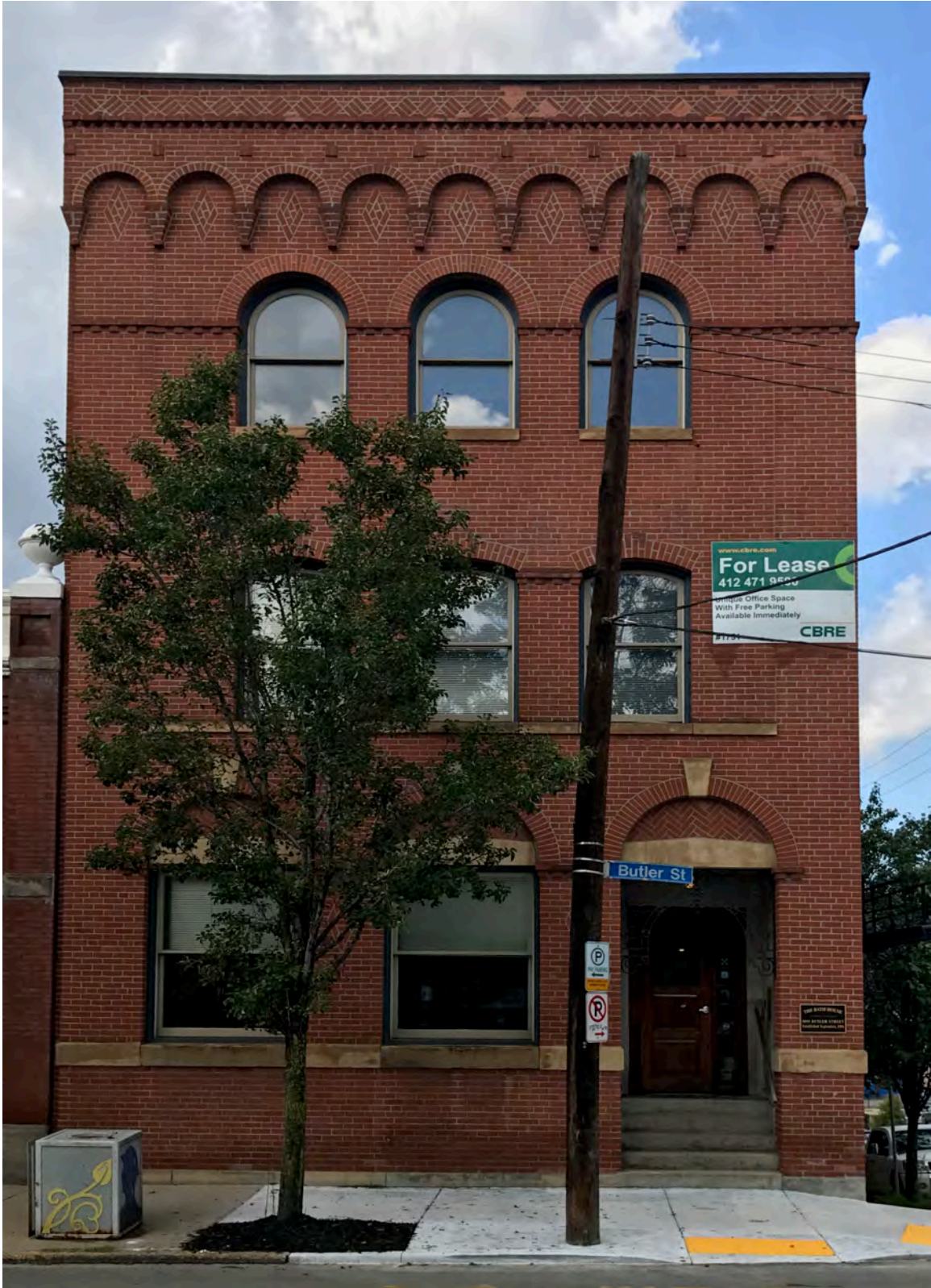
Photograph 2. Front Elevation (Butler Street).
