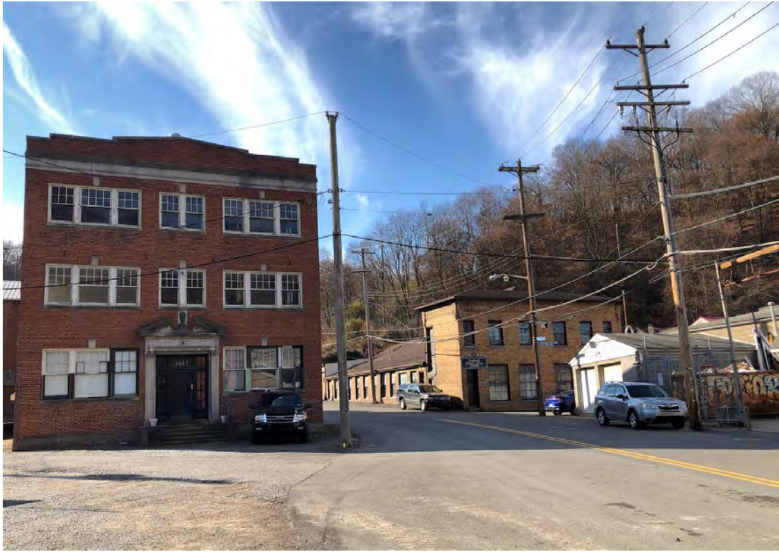
Photo 1. Streetscape, looking west, showing the buff brick front of 160 Warden Street (center right) with McCartney Street running along the building's south facade. The ca. 1930s red brick building (left) is listed on the 1950 Sanborn Map as "office and apartments" and for many decades was part of the holdings of Dacar Chemical Company.
