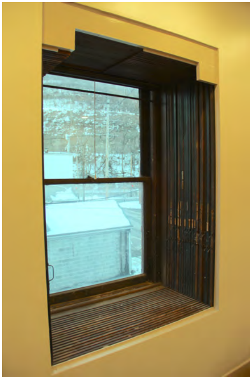
Photo 22. Display window, second-floor office space, looking southeast, showing the nineteen right-hand sliding display panels in their stored position within the wall (Preservation Pittsburgh).
