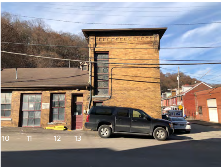
Photo 12. South facade, looking north, showing Bays 10 through 13 in the shed portion of the building along with the two-story headhouse to the right.
