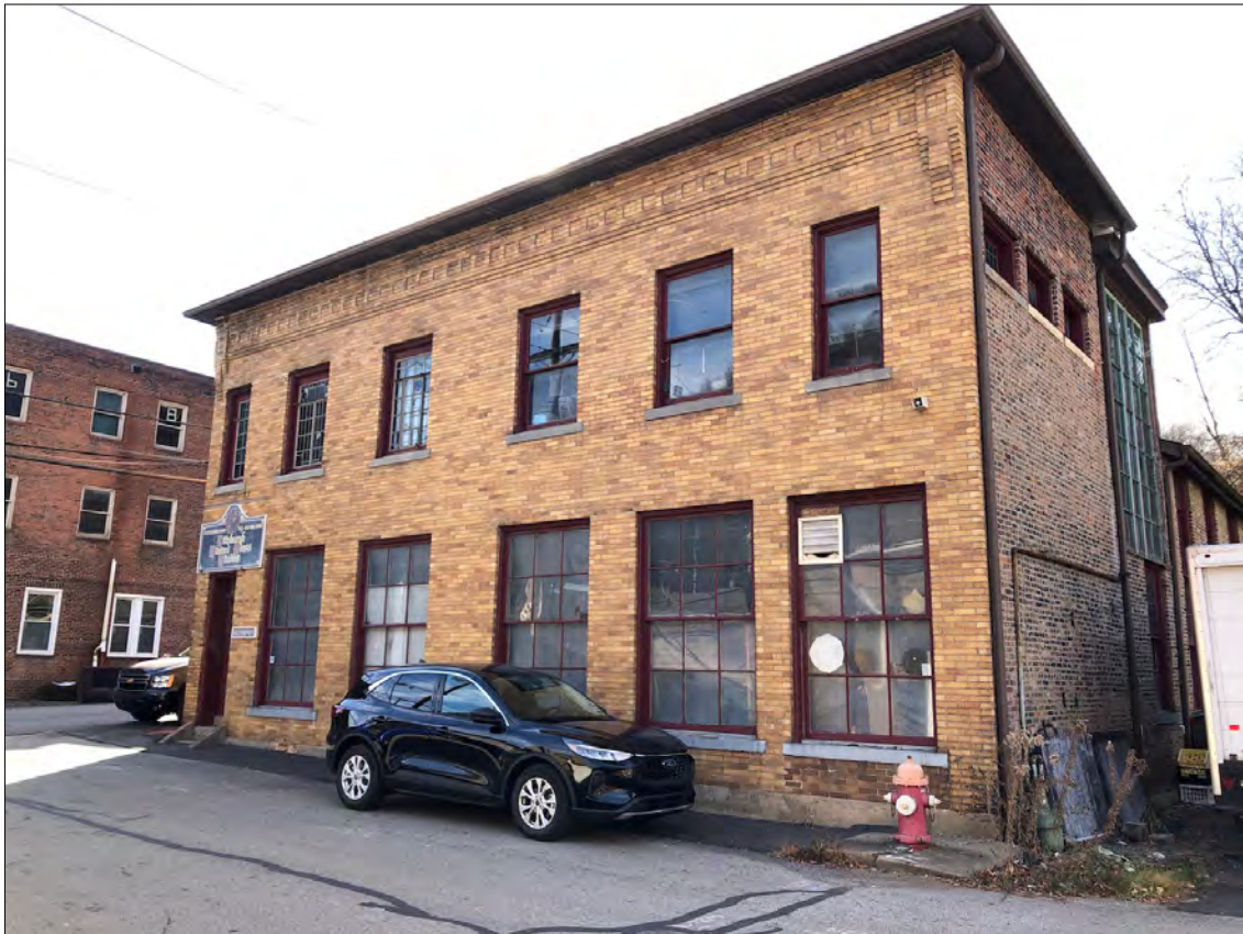
Photo 5. Front/east facade, looking southwest. The two different brick types used on the building are visible: buff-colored face brick on the front and more utilitarian common brick in reds and yellows on the north facade (right).
