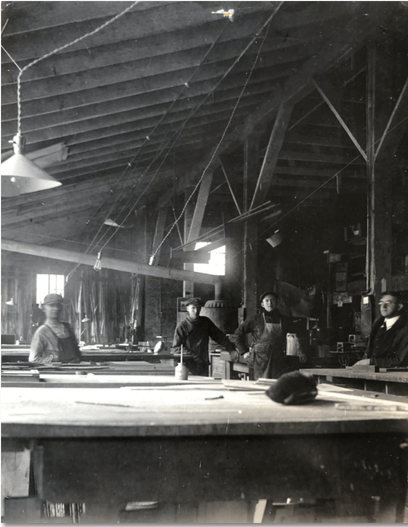
Figure 6 (left). Interior of the shed, looking west, ca. 1913 (soon after the building was first occupied by Pittsburgh Art Glass). Employees are gathered around work benches in the stained glass workshop. To the right is the double-height interior of the 1903 Wayman and Wood warehouse addition before the mezzanine was inserted in the 1920s. The two windows visible in the west wall would stop illuminated the space after the garage/loading dock is built in 1946 (Pittsburgh Stained Glass Studio Records).
