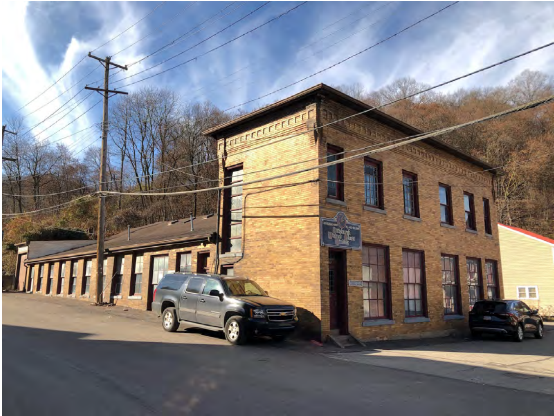
Photo 8. South facade (left) and front facade (right), looking northwest, showing the early-twentieth century “headhouse and shed” design.
