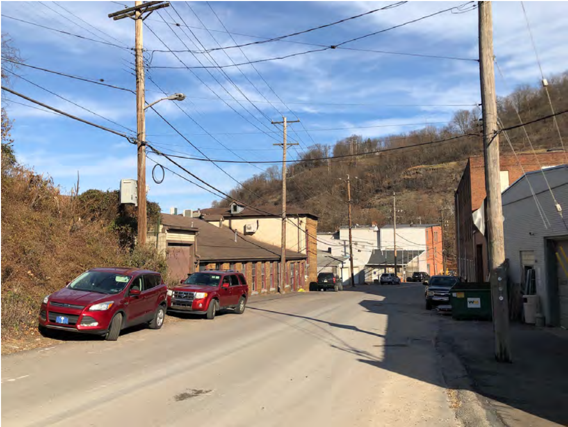
Photo 3. Streetscape, looking east, showing McCartney Street passing along the south side of the PSGS building.
