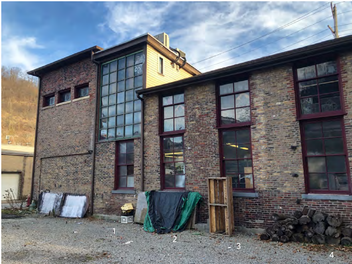
Photo 14. North facade, looking southeast, showing (from left to right) the headhouse, exhibition room and shed.
