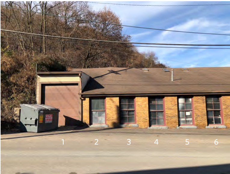
Photo 10. South facade, looking north, showing Bays 1 through 6 in the shed portion of the building.
