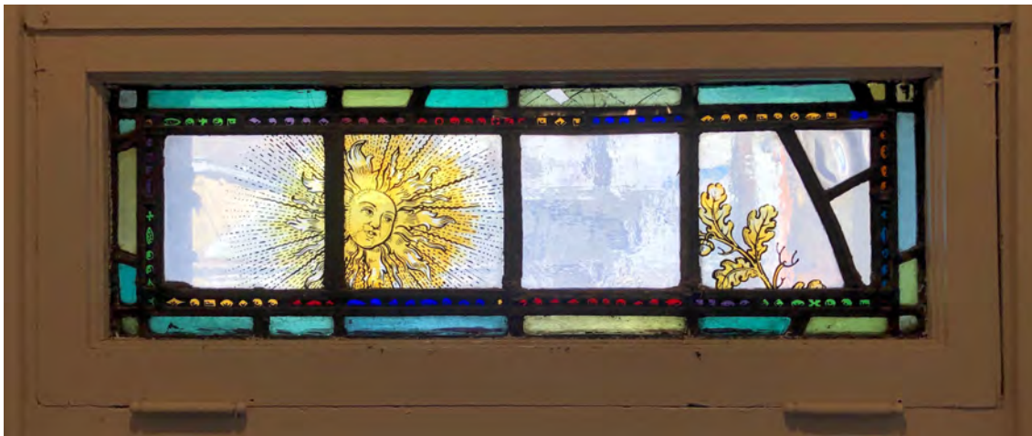
Photo 16. Transom above the front entry, looking east from the interior stairs.
