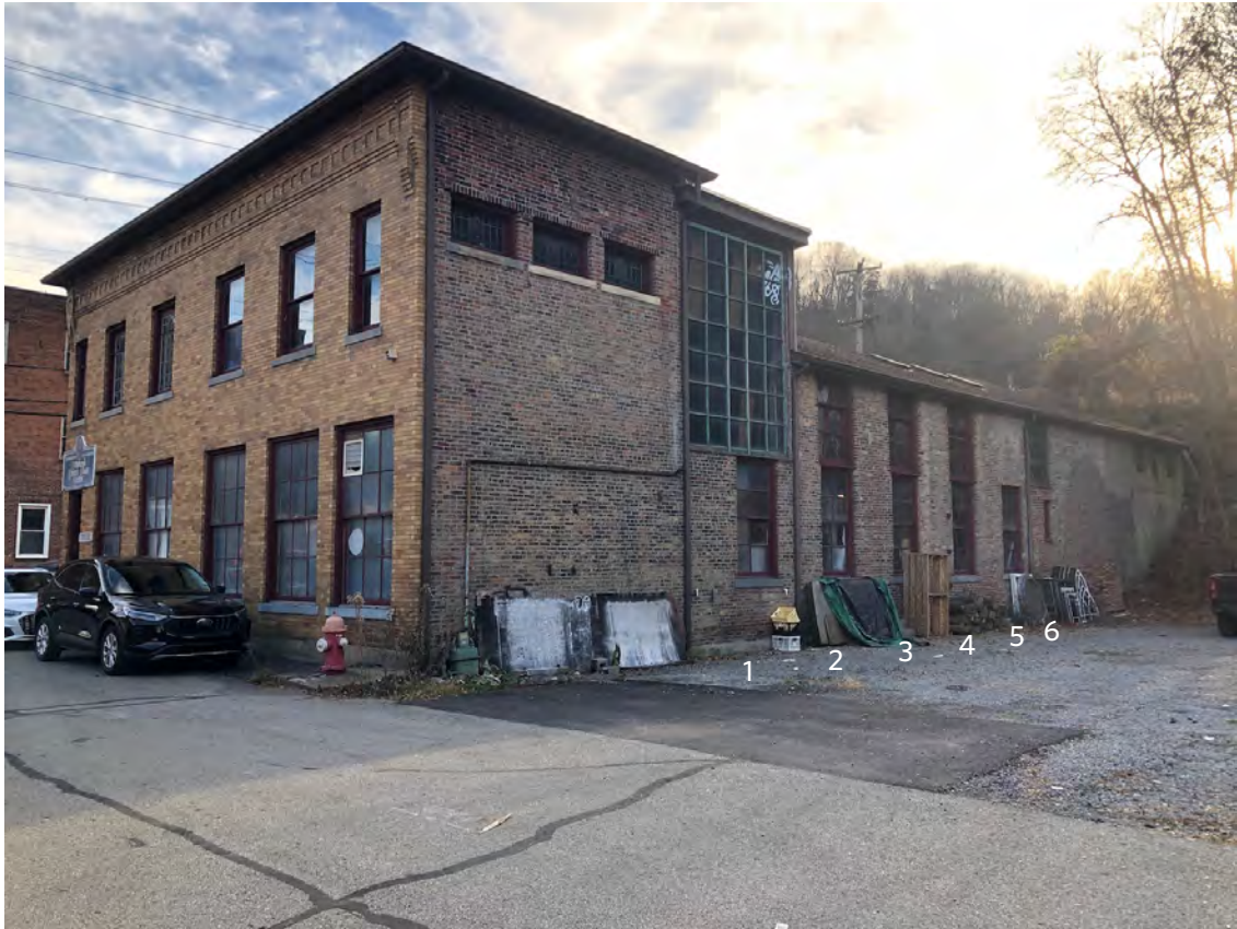
Photo 13. North facade (right), looking southwest, showing (from left to right) the headhouse, exhibition room and shed. Also shown are numbers identifying bays in this facade of the shed.
