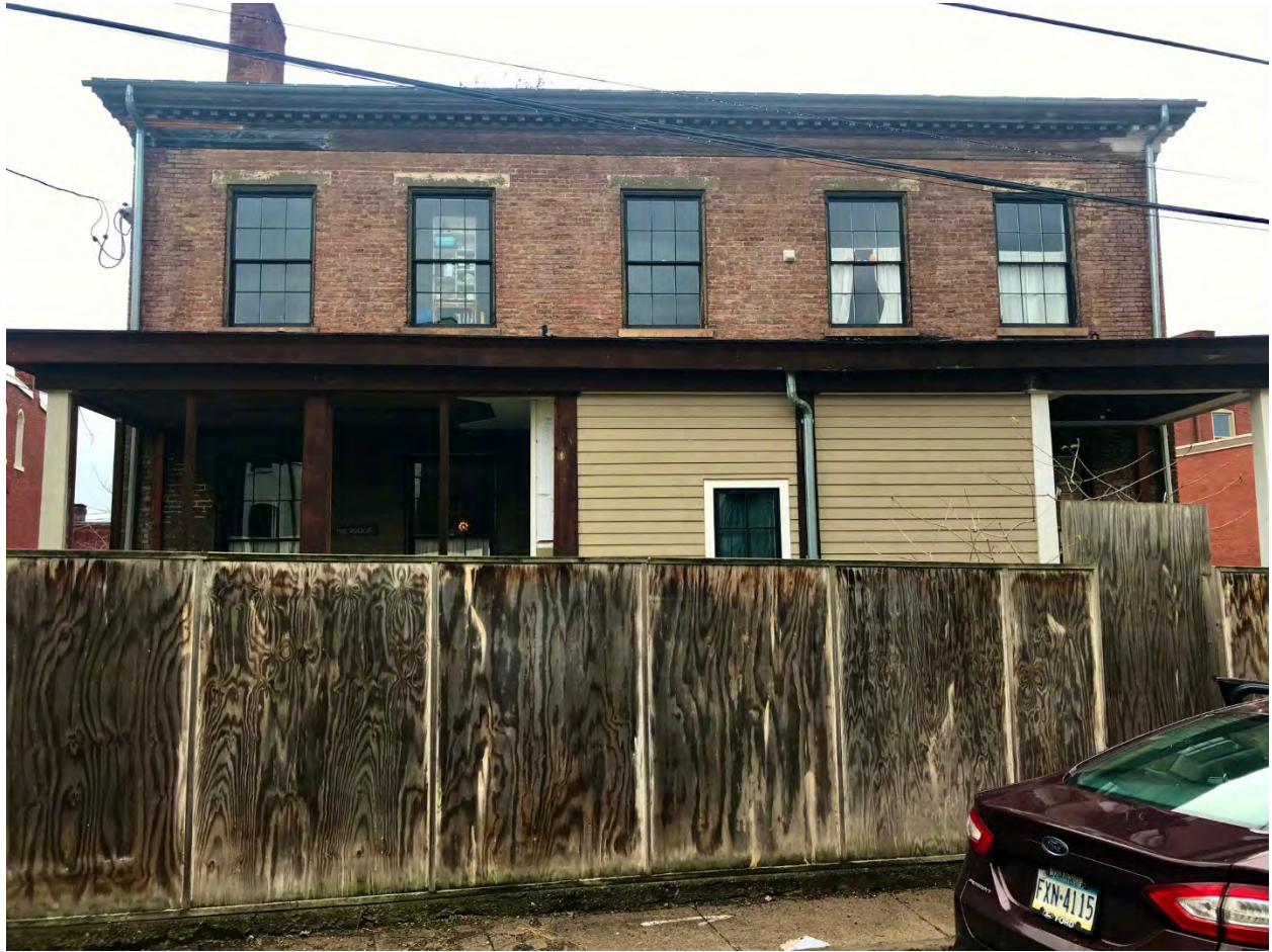
Photo 9. Echo , Rear Elevation, January 10, 2020. Source: Preservation Pittsburgh.
