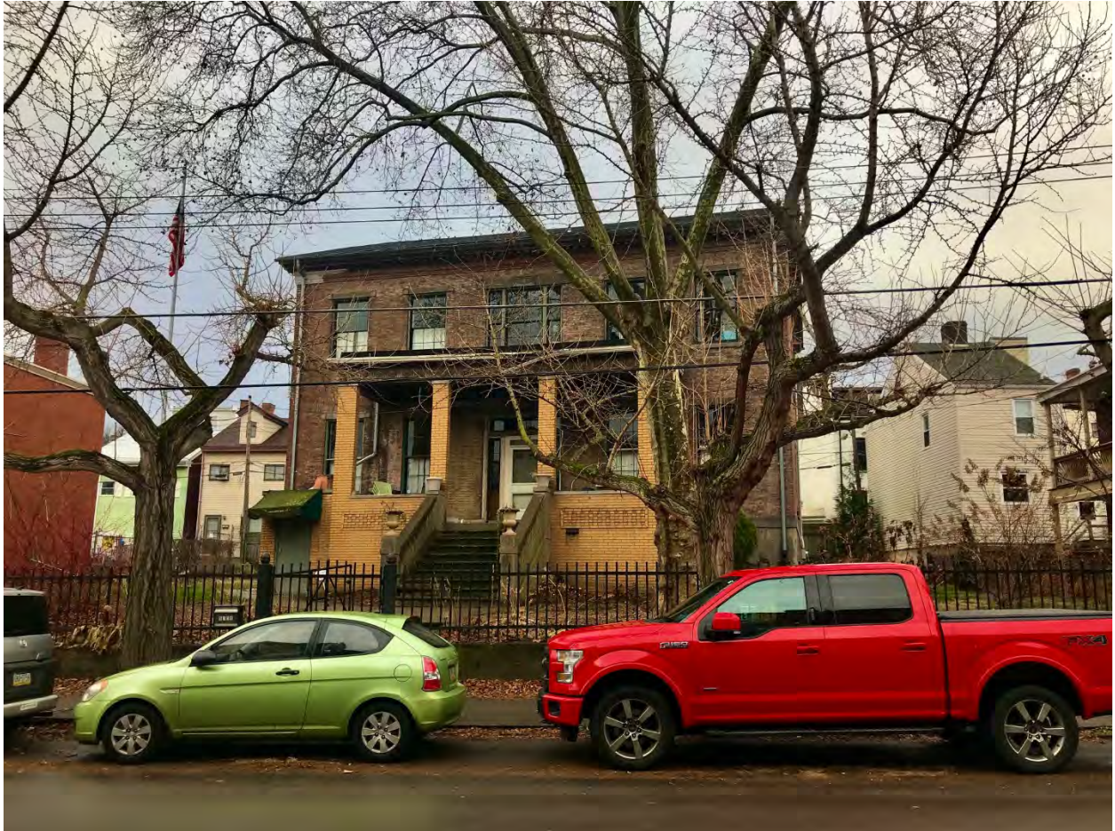
Photo. 1. Echo, Primary Façade . January 10, 2020. Source: Preservation Pittsburgh.
