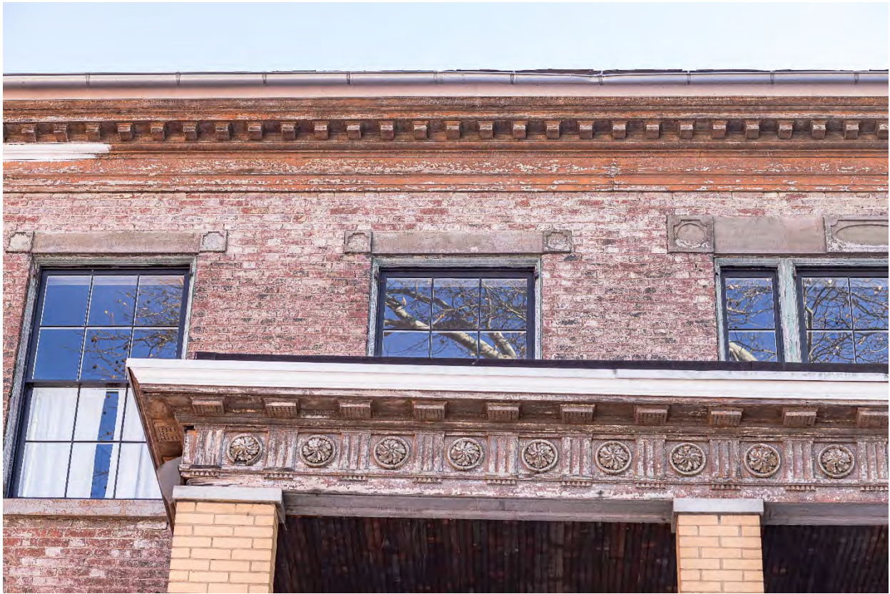
Photo. 5. Echo, Cornice & Freeze Detail , January 10, 2020. Source: Preservation Pittsburgh.
