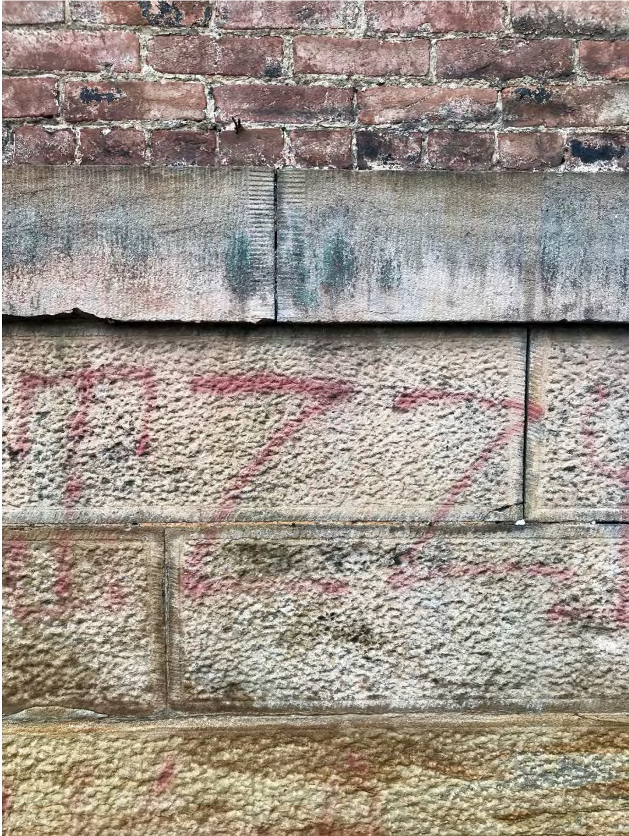
Photo. 3. Echo, Foundation and Brick Detail, South Elevation. January 10, 2020. Source: Preservation Pittsburgh.
