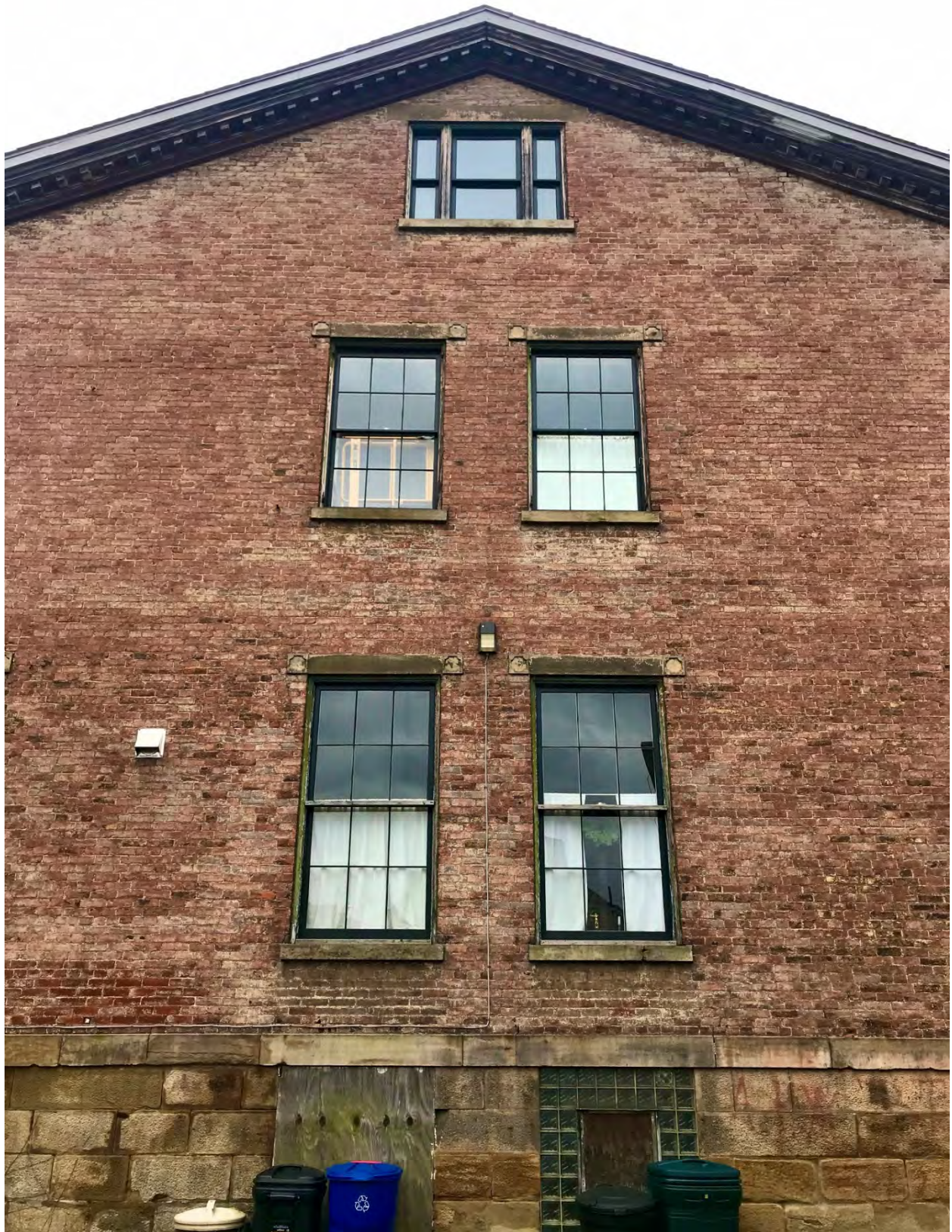
Photo. 12. Echo, South Elevation , January 10, 2020. Source: Preservation Pittsburgh.
