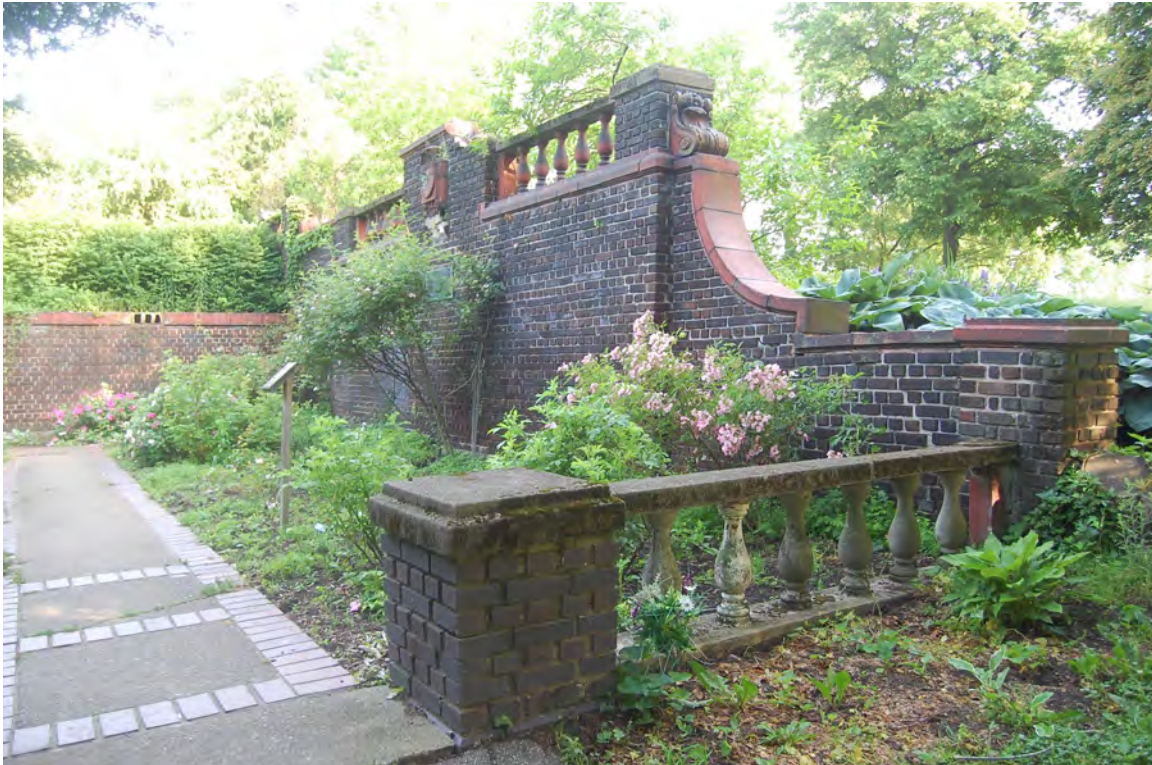
Photo 7. Terraced Garden, north side wall of lower terrace
