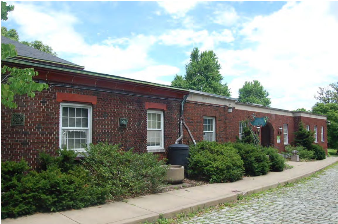
Photo 54. Side of Garden Center along Mellon Park Road. Change in brick color and cornice material mark transition from original garage to modern addition.
