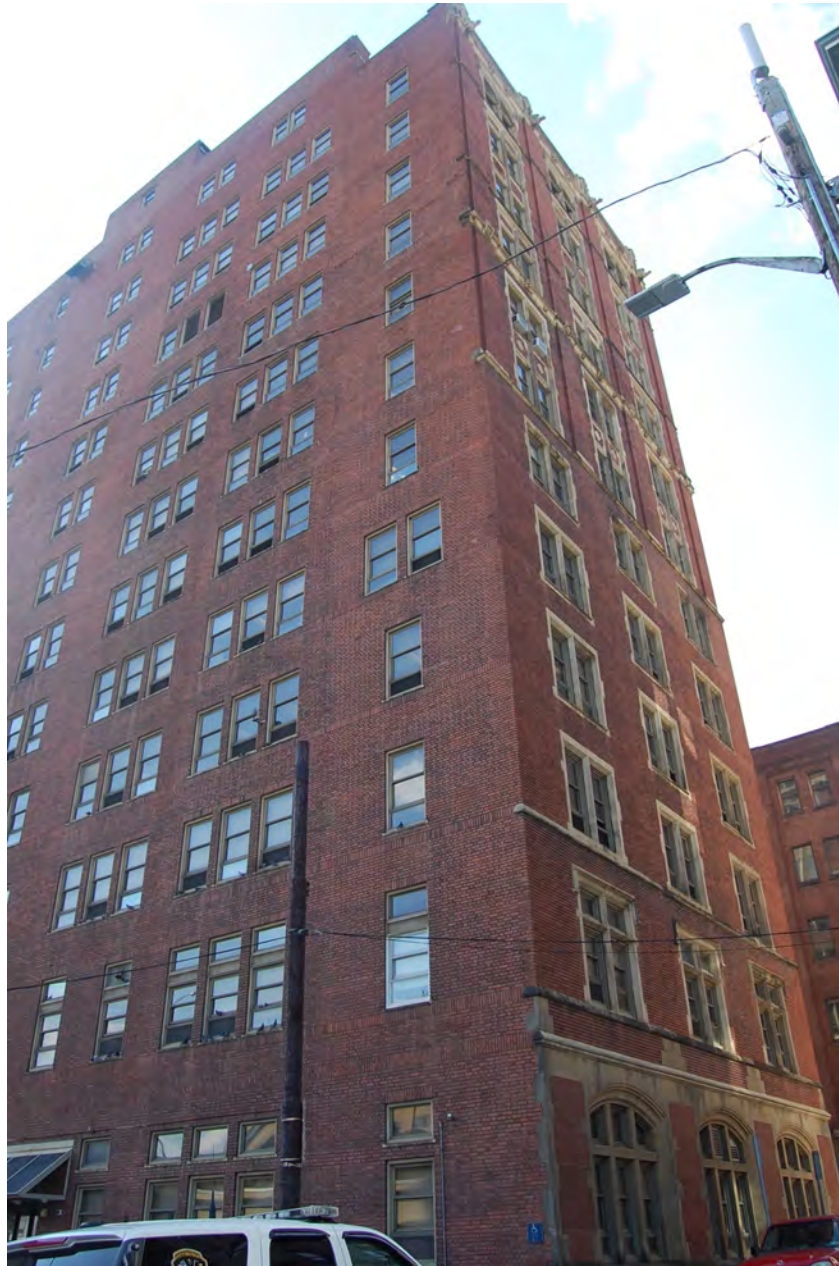
Photo 5. Former Jones & Laughlin Building (now John P. Robin Civic Building), 200 Ross Street, rear and north (Third Ave.) elevations
