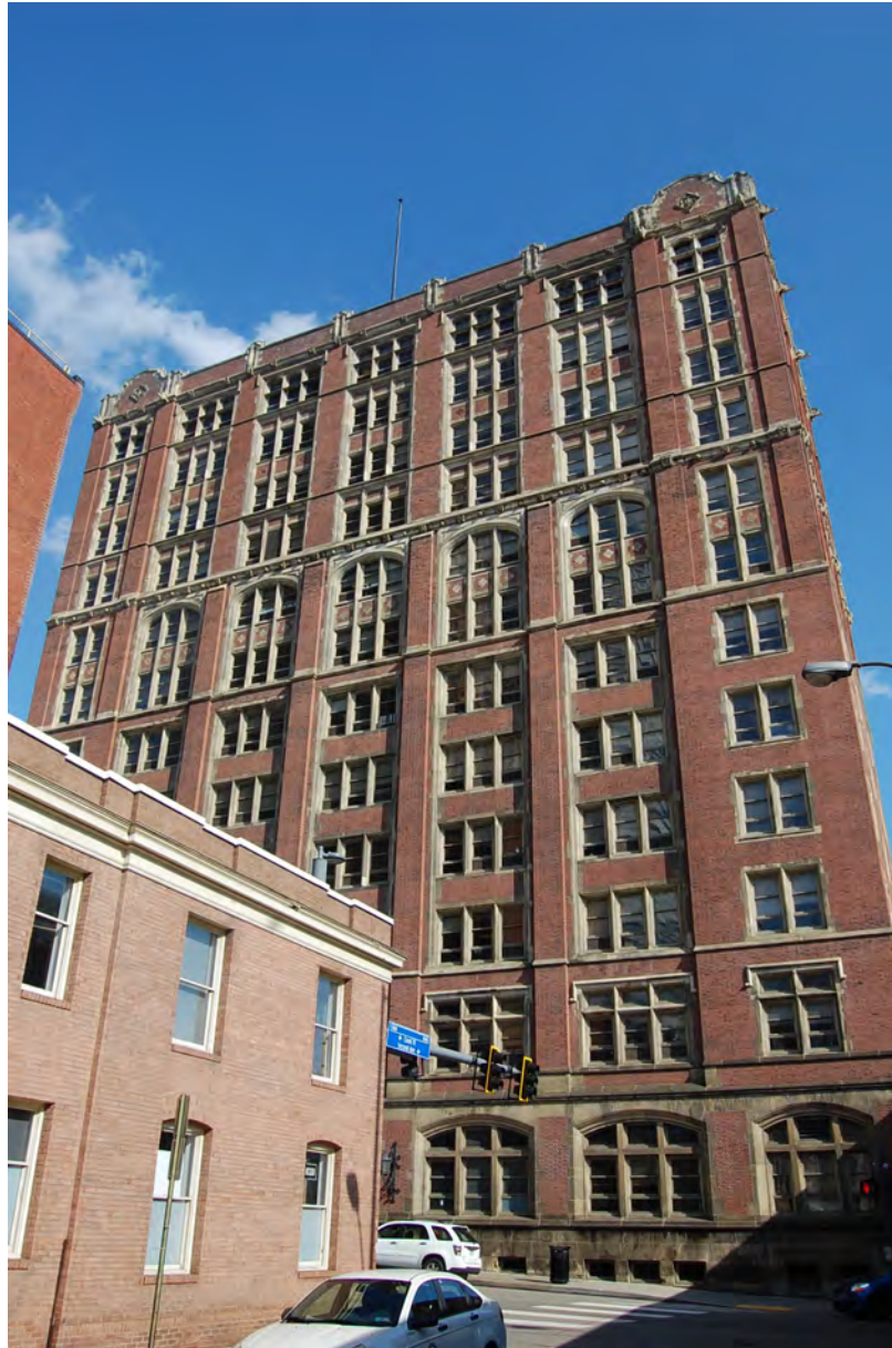
Photo 2. Former Jones & Laughlin Building (now John P. Robin Civic Building), 200 Ross Street, view from Second Ave.
