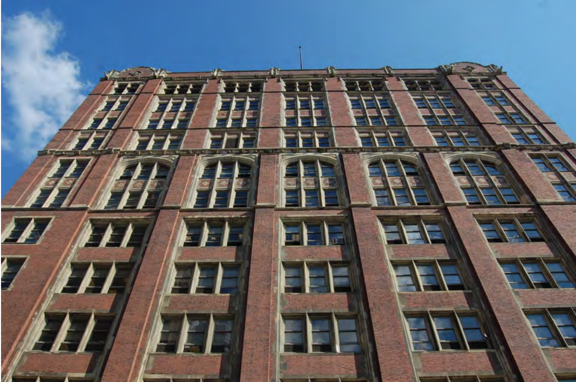
Photo 3. Former Jones & Laughlin Building (now John P. Robin Civic Building), 200 Ross Street, 4th-12th stories
