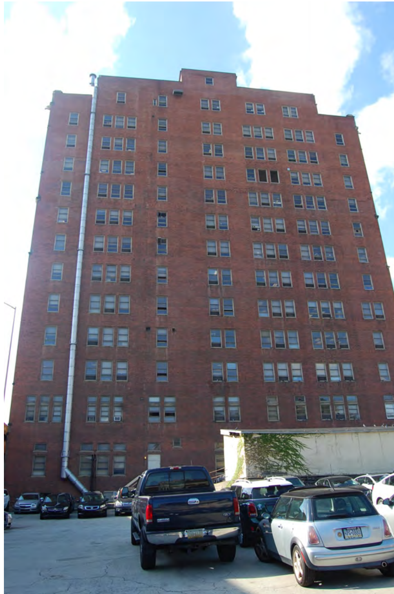
Photo 6. Former Jones & Laughlin Building (now John P. Robin Civic Building), 200 Ross Street, rear elevation from parking lot. The 13th floor is visible only from the rear.
