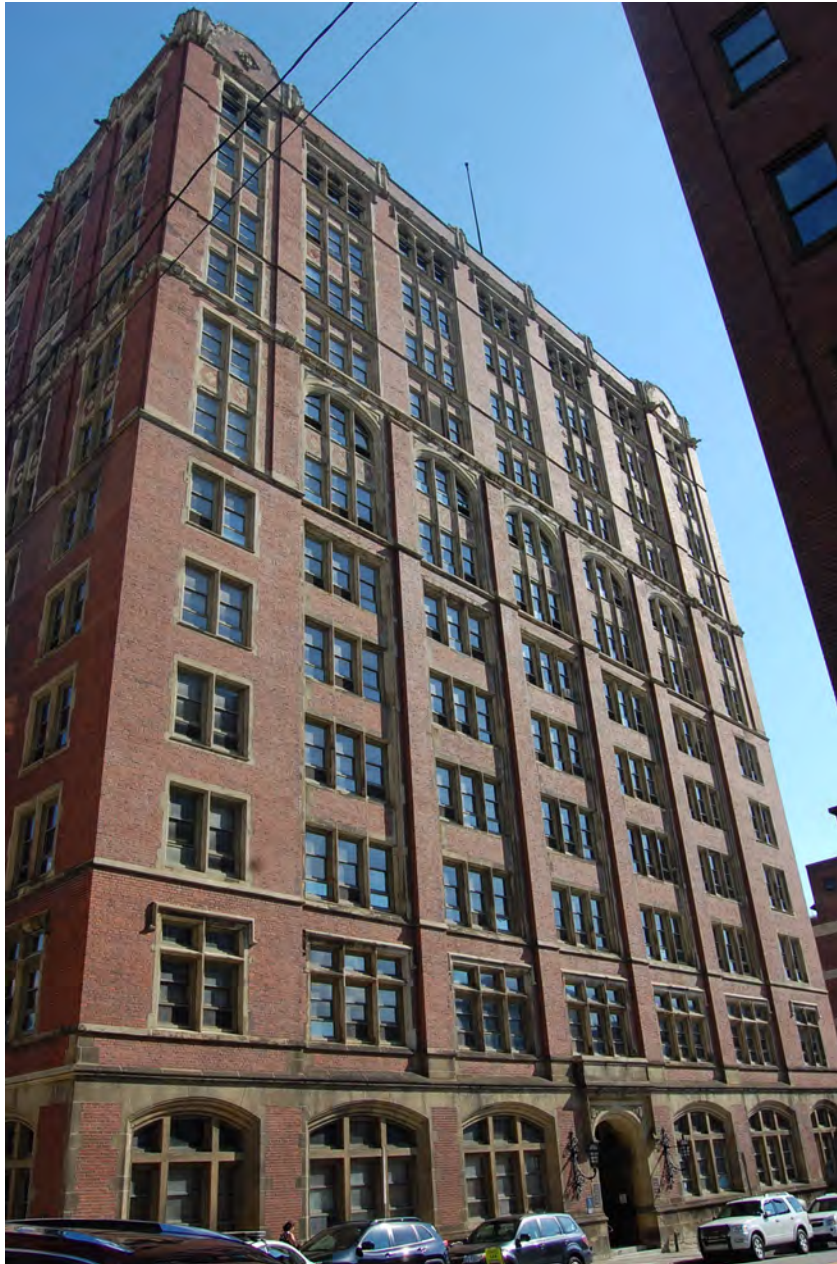
Photo 1. Former Jones & Laughlin Building (now John P. Robin Civic Building), 200 Ross Street, view from Third Ave.
