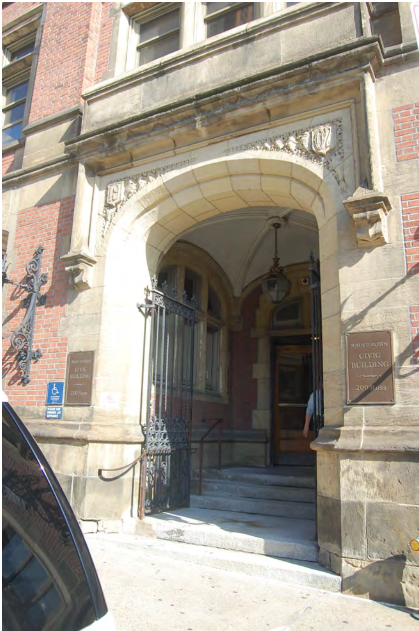
Photo 7. Former Jones & Laughlin Building (now John P. Robin Civic Building), 200 Ross Street, main entrance
