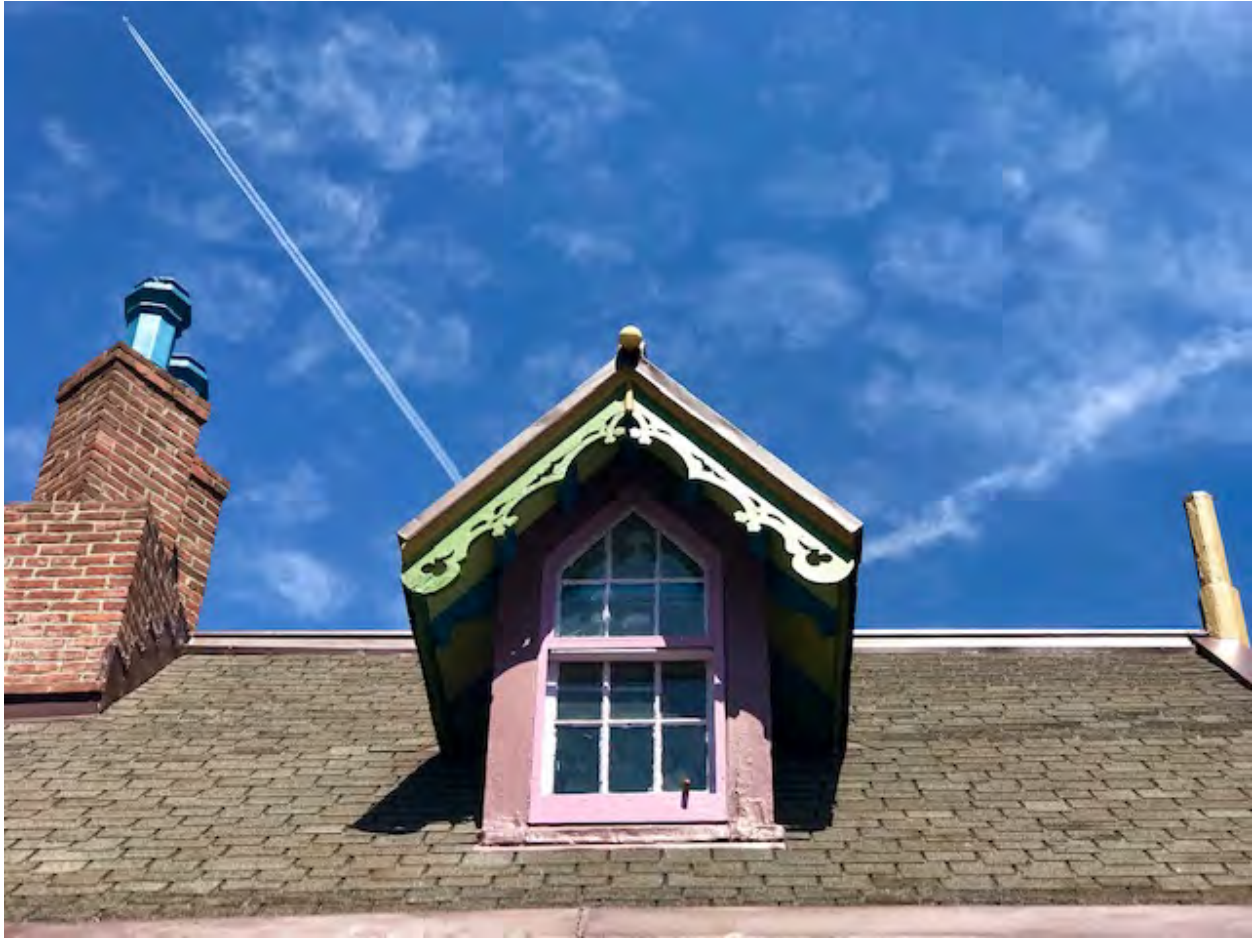
Photo. 9. Heathside Cottage, Eastern Wing, Dormer Detail , April 2019. Source: Matthew W.C. Falcone.
