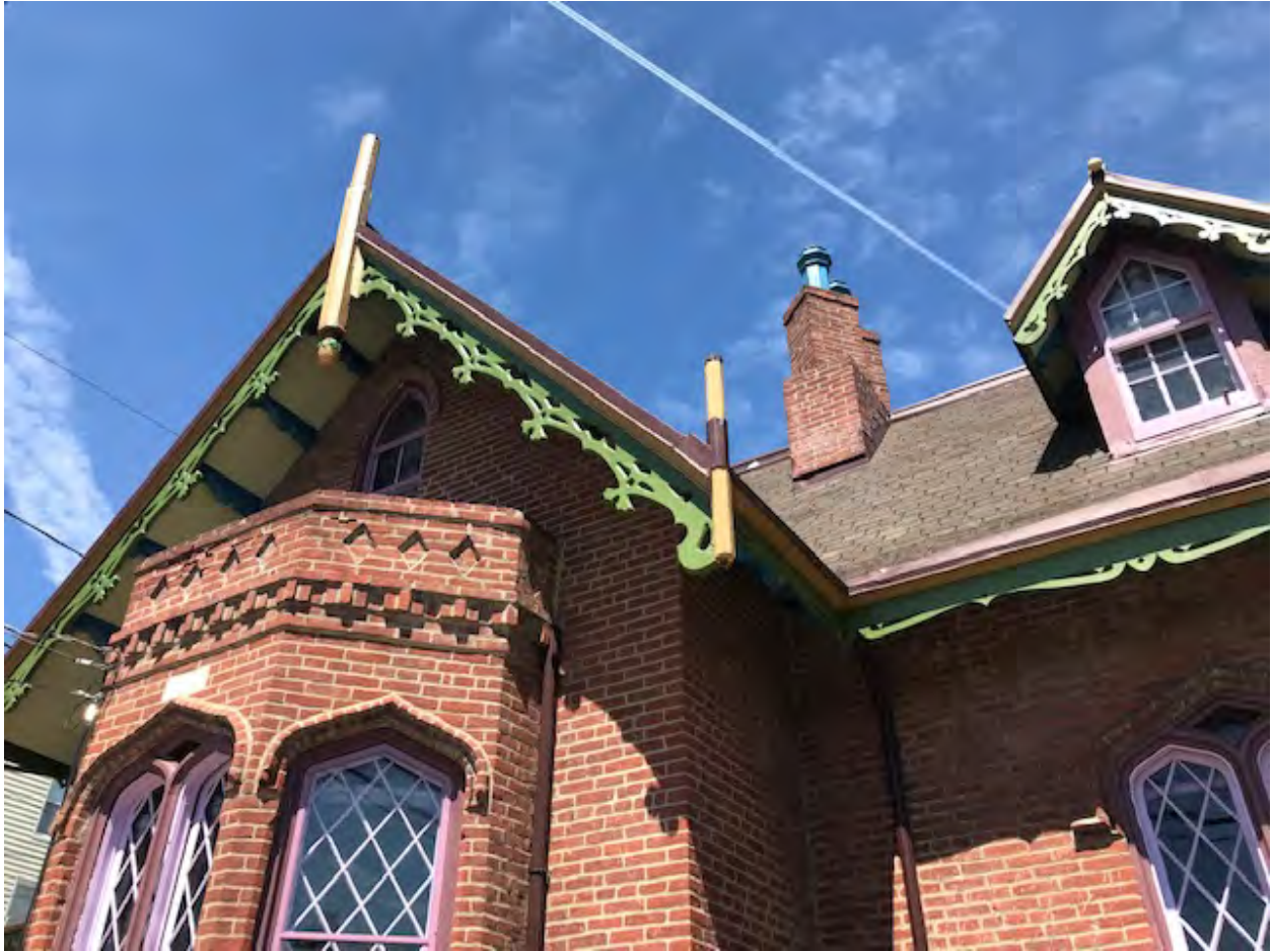
Photo. 4. Heathside Cottage, Bargeboard and Roof Detail , April 2019. Source: Matthew W.C. Falcone.
