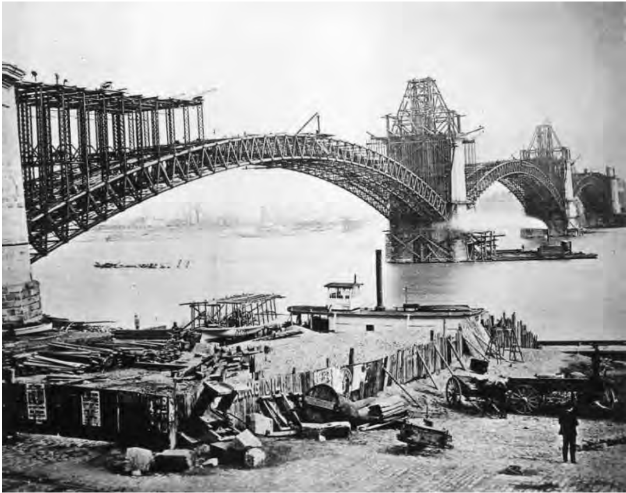
Eads Bridge Under Construction, 1870. Library of Congress.
