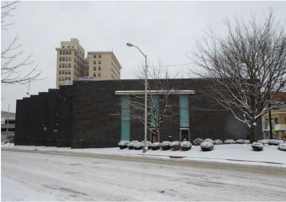
Figure 3: Mellon National Bank, East Liberty Office, showing southeast (side) facade, facing northwest (Mary Barenfeld).
