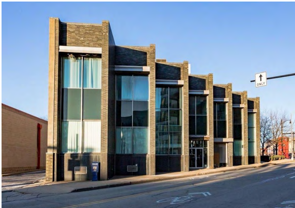
Figure 5: Mellon National Bank, East Liberty Office, showing southwest (rear) facade, facing northeast (Amy Fisher).
