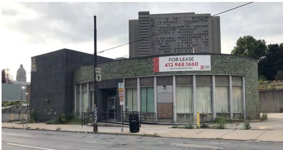
Figure 20: Upper Fifth branch. Location: 1425 Fifth Avenue, Pittsburgh PA 15219. Current Use: Vacant. Source: Brittany Reilly, August 2020.
