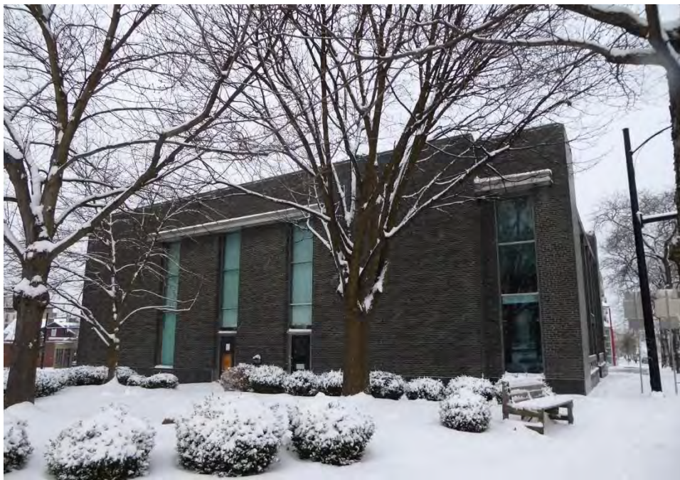
Figure 2: Mellon National Bank, East Liberty Office, showing southeast (side) facade, facing southwest (Mary Barendsfeld).
