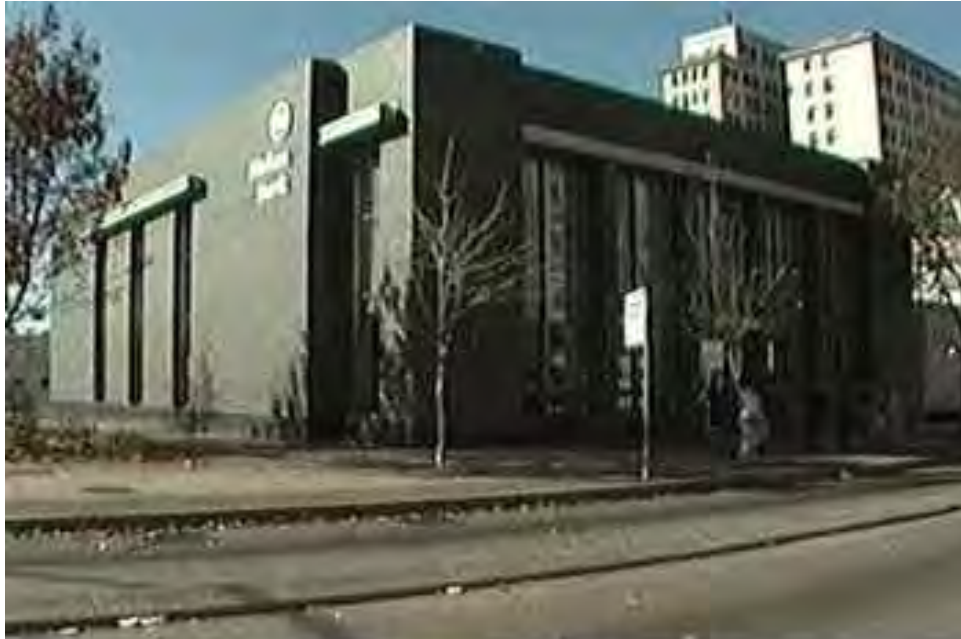
Figure 18: 6112 Penn Avenue. Allegheny County Real Estate Portal. Photographer and date unknown (post 1971).
