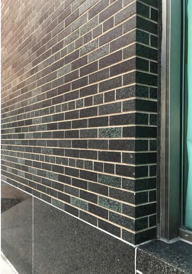
Figure 9: Mellon National Bank, East Liberty Office, detail view showing glazed brick and terrazzo cladding, facing southwest (Brittany Reilly).
