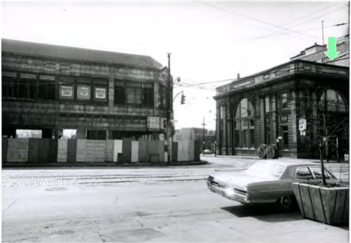
Figure 15: Penn and Centre Avenues During Renewal. Historic Pittsburgh, Melvin Seidenberg Photographs. Photographer: Coughanour, Harry, Jr, Urban Redevelopment Authority. Date: March 12, 1967.
