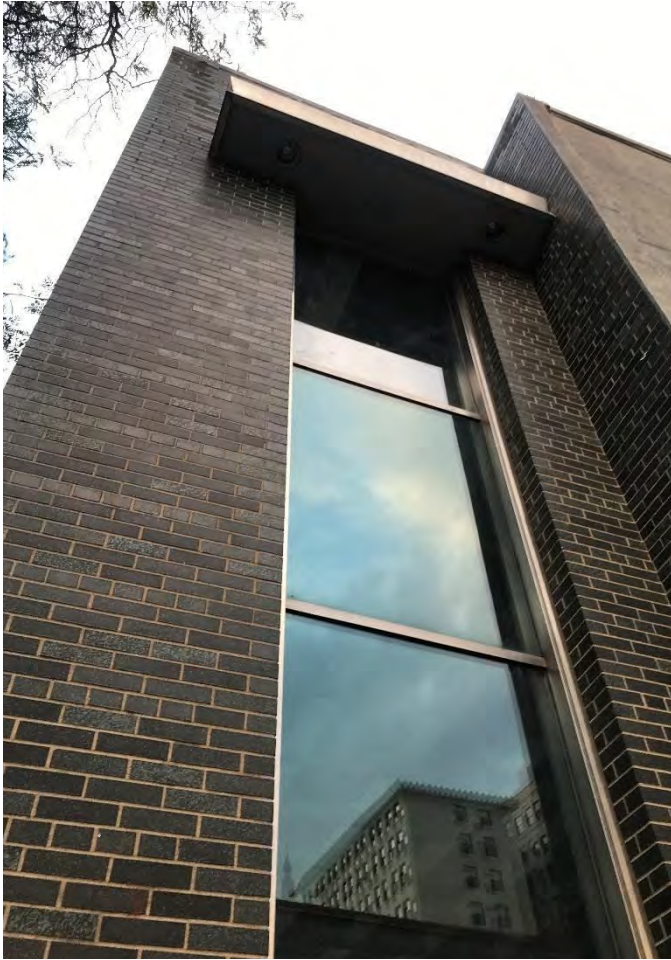
Figure 11: Mellon National Bank, East Liberty Office, detail view showing wall, glazing, and aluminum fascia on northwest (side) facade, facing southeast (Brittany Reilly).
