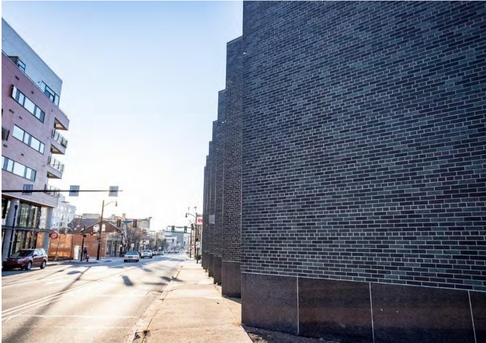
Figure 8: Mellon National Bank, East Liberty Office, detail view showing glazed brick and terrazzo cladding, facing southwest (Amy Fisher).
