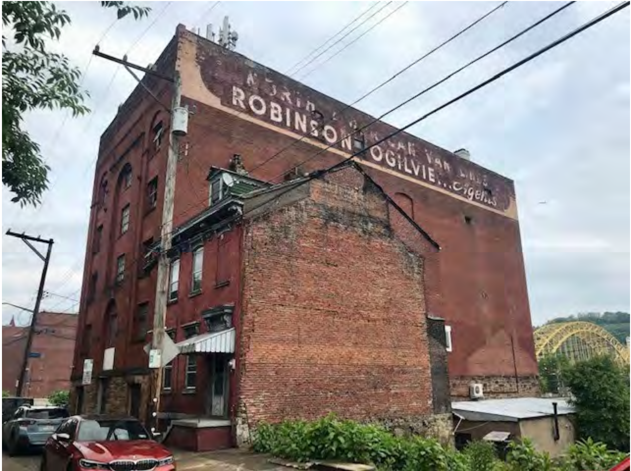
Photo. 1. Primary & Western Tertiary Façades, 855 S. Canal Street. Matthew Falcone. May 2023.
