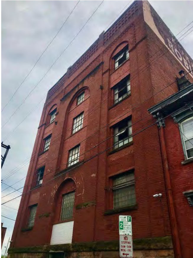
Photo. 2. Primary Façade, 855 S. Canal Street. Matthew Falcone. May 2023.
